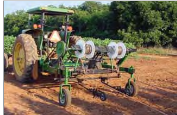
System used to install surface drip tape.
